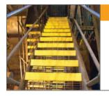
Long wearing, anti-corrosive, non-slip nosing designed to re-profile the leading edge of any step are the characteristics of StairSAFE™
